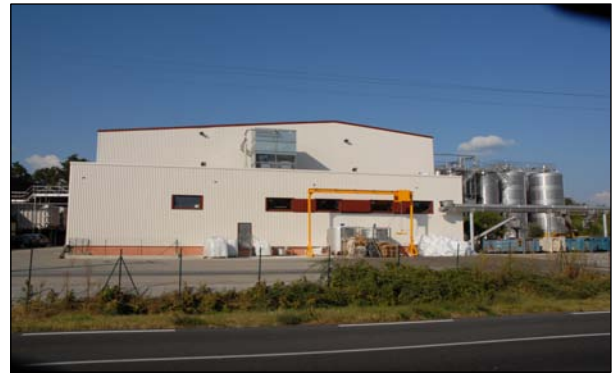
Cave Coopérative de Routier (Aude) : re-organization of the wine-making facility vinification.
